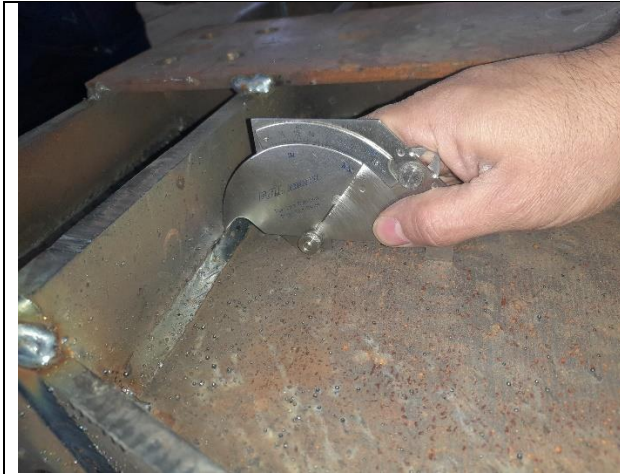
9. Weld Check by Cambridge Gage
