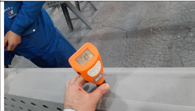
Sandblasting surface roughness control
