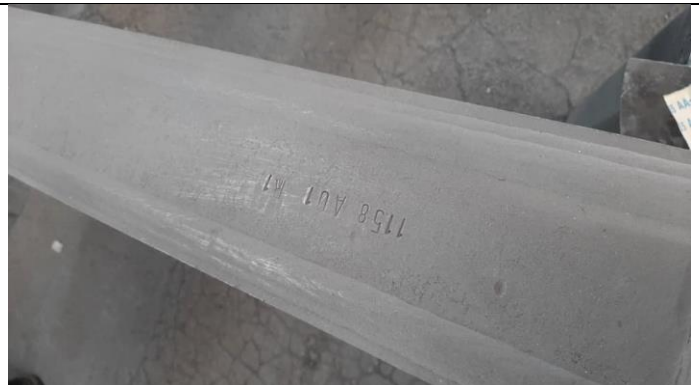
Visual control of sandblasting surface
