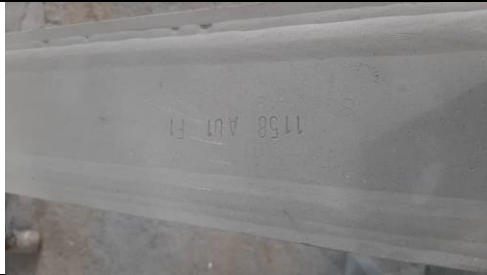
Visual control of sandblasting surface
