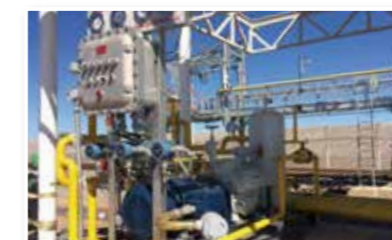
LPG transfer compressor - Mexico 6HK / 45kW
