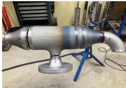
Piping fitted ready for inspection
